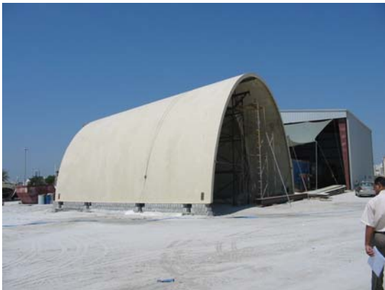
Figure 7(a) Panels on the Assembly Jig
