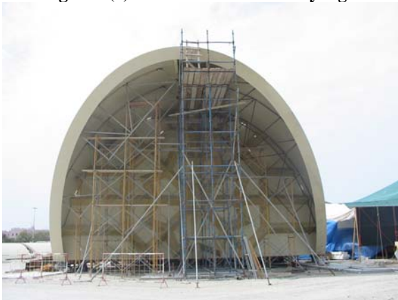
Figure 7 (b) Front Fascia Panel Assembly
