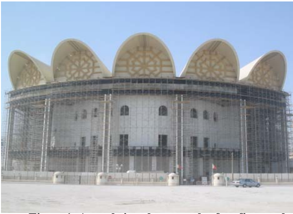
Figure 1. Actual site photograph after five vaults are installed
