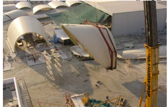
Figure 8 (b) – Front Section lifting on jig
