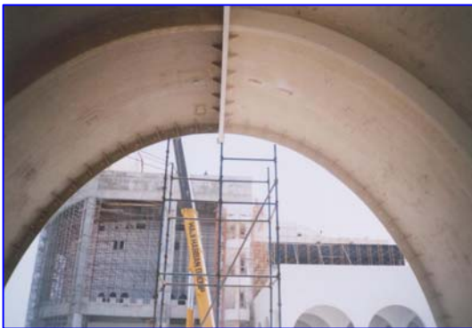
Figure 7 (c) Ridge Flange Bolting
