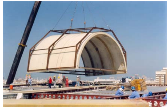
Figure 8 (a) – Central Section lifting on jig
