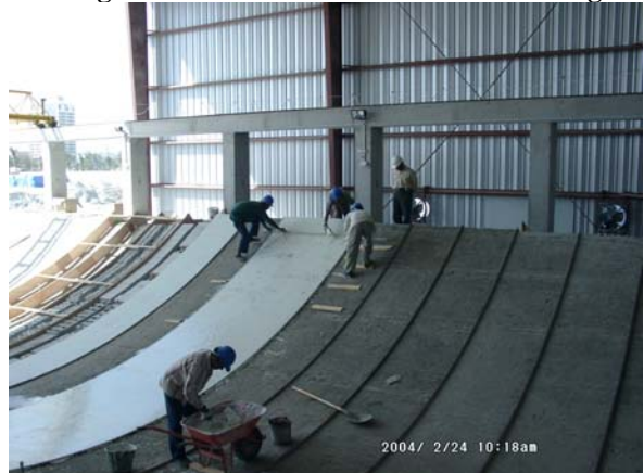
Figure 4b- Mould under Construction Stage 2
