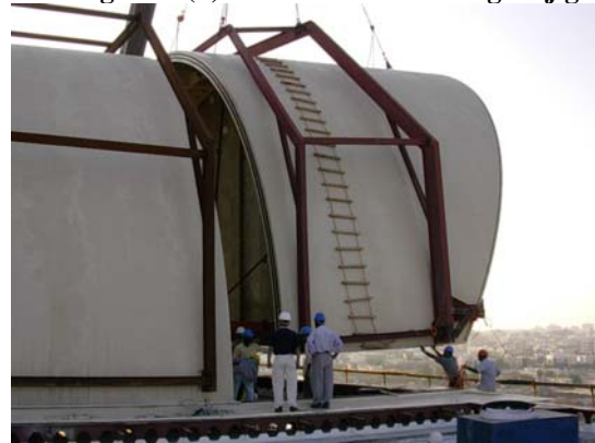
Figure 8 (c) – Front & Central section alignment
