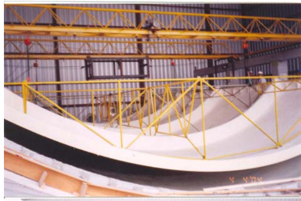
Figure 5 (b)- Jigs for demolding and handling.
