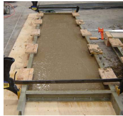
Figure – 5. Formwork for concrete specimens with wet concrete prior to setting (Specimen 4).
