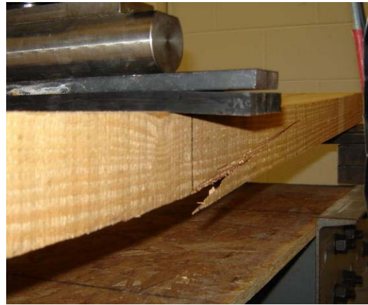
Figure – 20. Bending tension failure seen in timber (Specimen 8).
