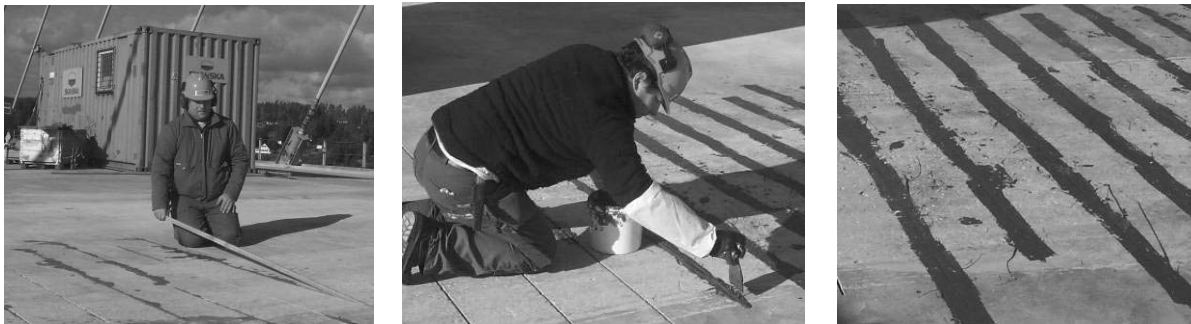
Figure 2: First NSMR field application in Sweden
